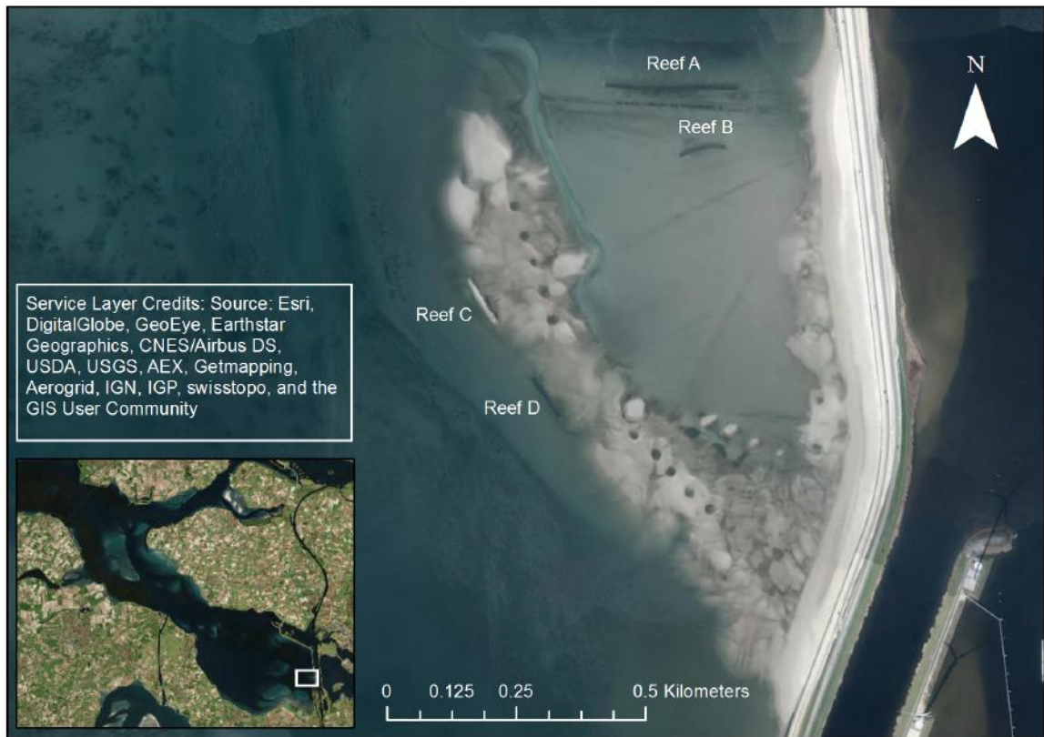
FIGURE 2.10: OESTERDAM NOURISHMENT LOCATION AND LAYOUT, WITH CONSTRUCTED OYSTER REEFS.
