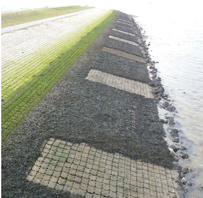
Fig. 19. The dike at Sint-Annaland after treatment with a bush trimmer (February 2017). Photo: T. van Oijen.
