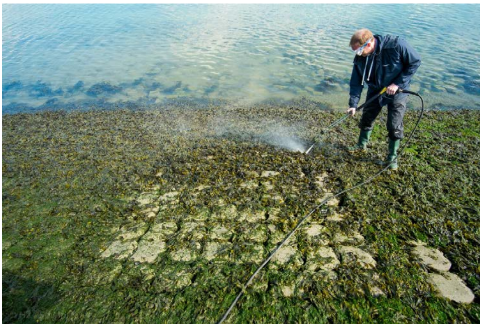
Figure 18. Treatment of dike sections with a power washer. Photo: E. Paree.
