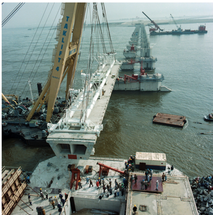
Figure 3 Reference design, Eastern Scheldt storm surge barrier [source: www.beeldbank.rws.nl ]
