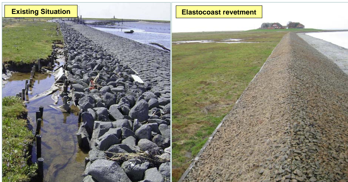
Figure 6-1: Existing situation and Elastocoast revetment on the Hallig Langeness (Photos: LKN)
