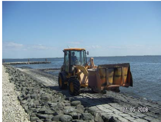
The rocks are tumbled with the polyurethane and transported to the construction site
