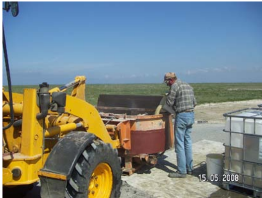
The polyurethane is added to the mixer
