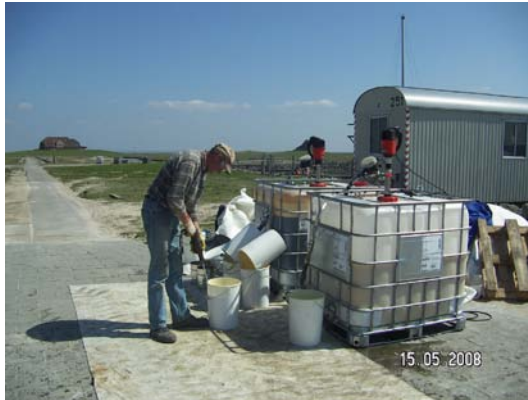
The polyurethane is filled into containers
