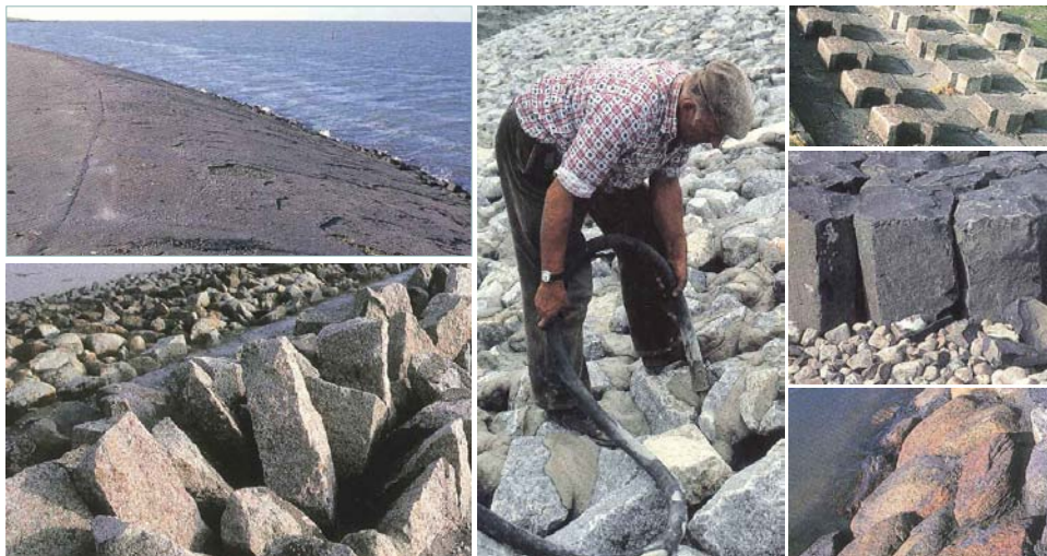
Figure 3-3: Design alternatives for revetments on the coastline
