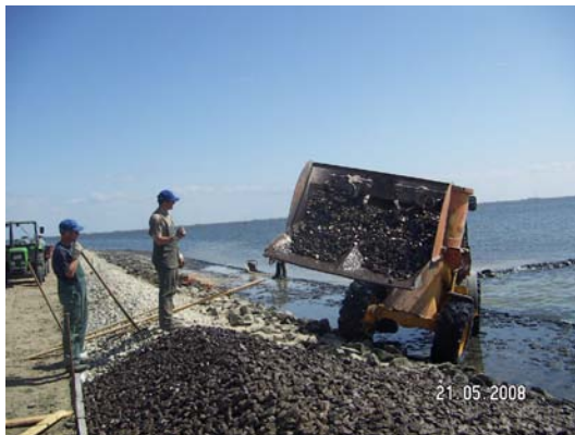
Installation at the construction site
