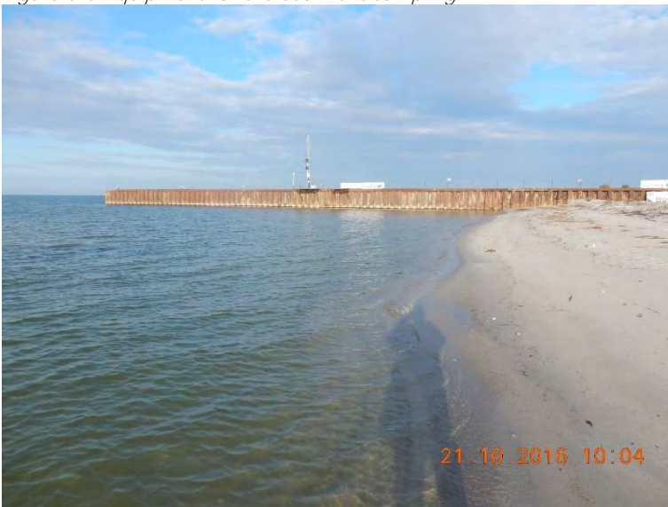
Figure 0-6 The water line and in the background the sheet-pile wall is observed
