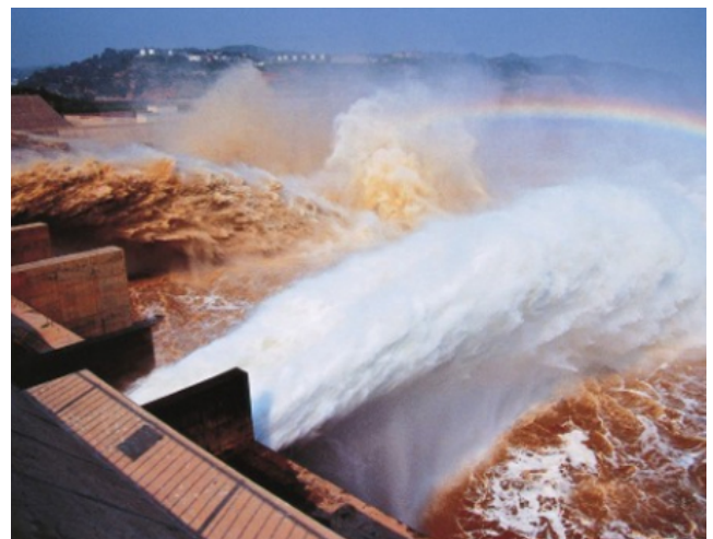
Figure 7: Man-made flood generation in the Yellow River at Xiaolangdi, China. The highly sediment-laden flow scours the river channel over a long distance downstream
