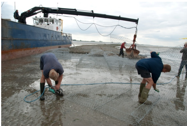
Figure 15: Placement of gabions with oyster shells (courtesy Tom Ysebaert)
