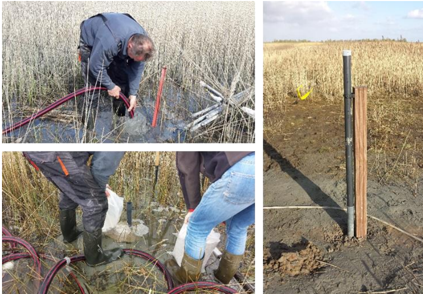
Figure 16. Installation of piezometers in tidal area using the flushing method.
