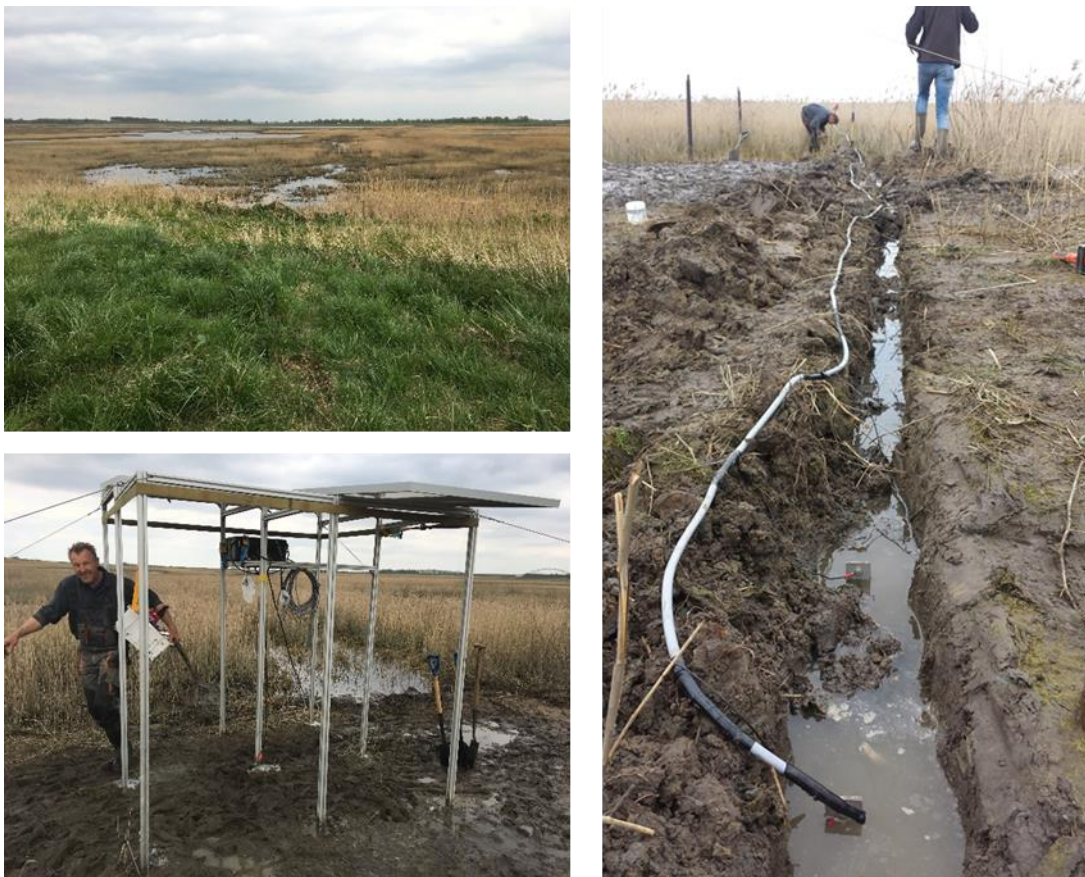
Figure 20. Installation of solar platform and ERT-cable in tidal area Rammegors.
