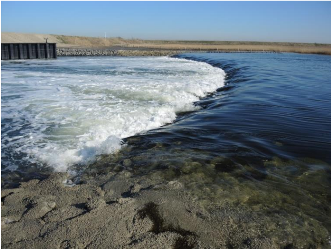
Figure 3. Outflow of saltwater during ebb from the Rammegors (right side of photo) into the Eastern Scheldt through the culverts in the Krabbenkreek dam (left side of photo). Photo: Tom Ysebaert.
